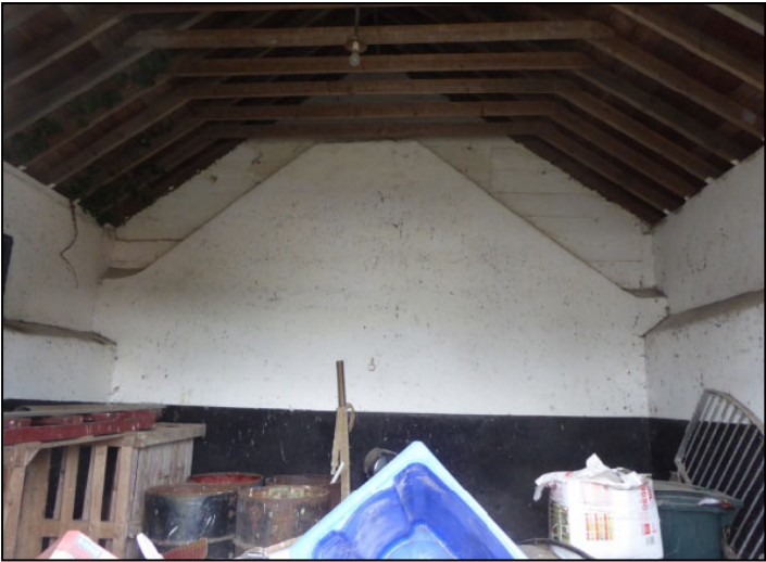
View inside the shed with the raised roof
